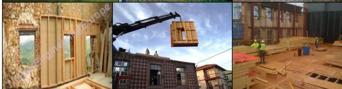
Load bearing insulated walls used in restorations. Traditional exterior with a 21st century interior
